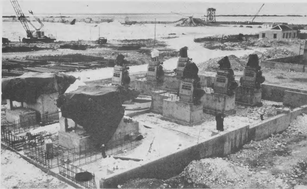
EARLY STAGES of construction of the ACI fertilizer works dot the area west of the Antilles ammonia plant. Prominent among the building is the compressor house, above, for the urea plant. In the far background is the lagoon and the workings involved in pier and dockside construction.
